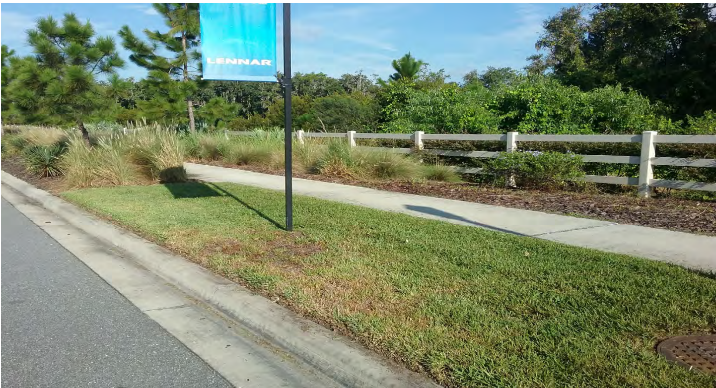
There are some voids along the fence where dead plants were removed that should be filled in.
